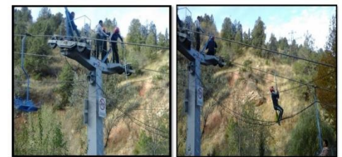
Picture: 5. Installation hinged ladders to the carrying rope.
