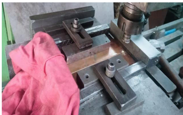
Fig-4: plates after clamping for welding.
