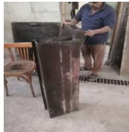
Figure 1.3: preparing of steel formwork.
