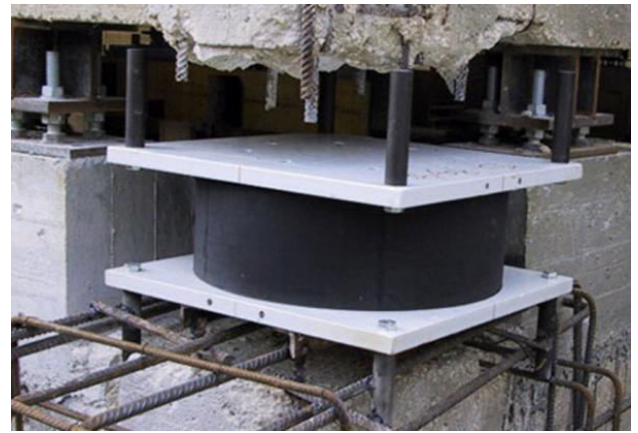
Fig 1.6: lead rubber bearing arrangement
