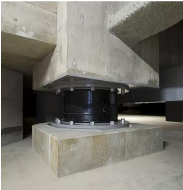
Fig 1.2: base isolation arrangement
