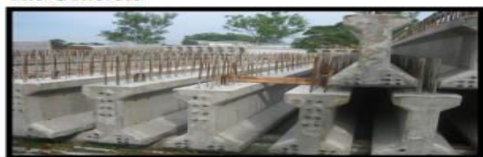
Concrete Will Be Cast Around The Ducts For Placing The Tendons
