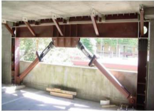
Arrangement of dampers in a building
