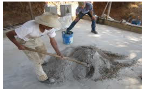
Fig (1.1): manual concrete mixing
