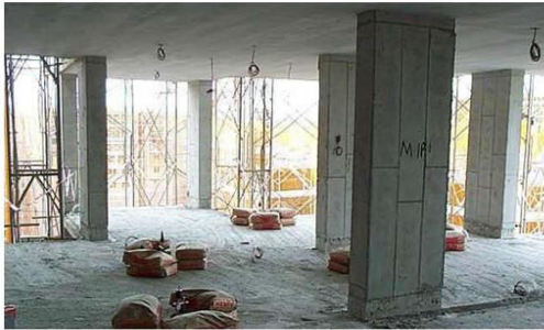
Fig 1.1 Flat Slab resting directly on columns
