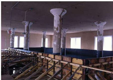
Fig 1.3 Flat slab with column capital
