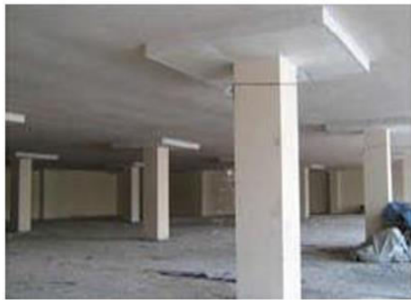
Fig 1.2 Flat Slab with Drop panels
