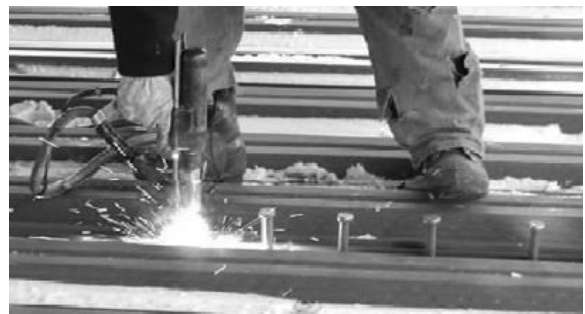
Figure 1: Shear Connectors
