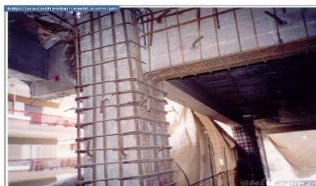
Fig: Concrete Jackting
