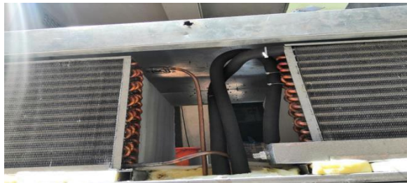
Figure: Copper pipe welding.
