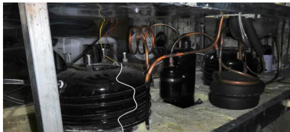
Figure: Copper pipe welding.
