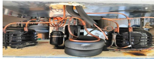
Figure: Refrigerant filling.
