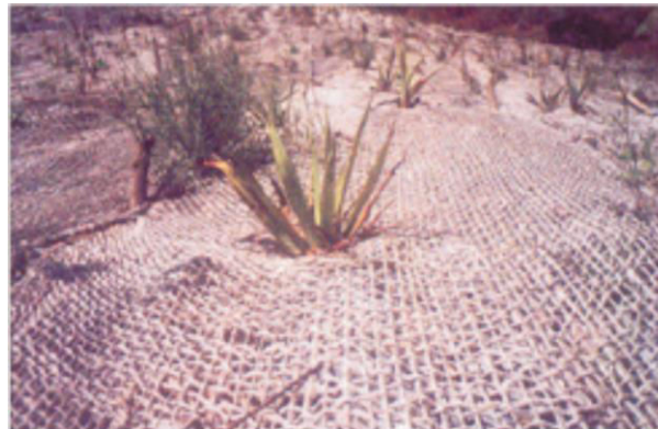
Fig 2.7 Growth of vegetation on slopes covered with jute geotextiles
