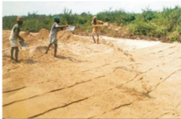
Fig 2.6 Laying of Jute Geotextiles for ground improvement
