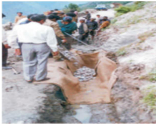
Fig 2.8 Laying of Jute geotxtileas Trench Drain
