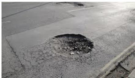
Figure 1.2: Pothole
