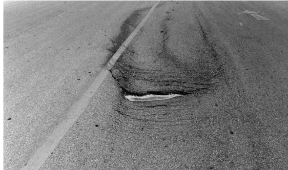
Figure 1.1: Slippage Crack
