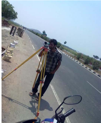
Fig 2.1 Surveying using dumpy level
