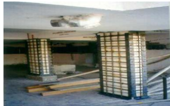
Fig. 2.1: Retrofitting using steel jacketing
