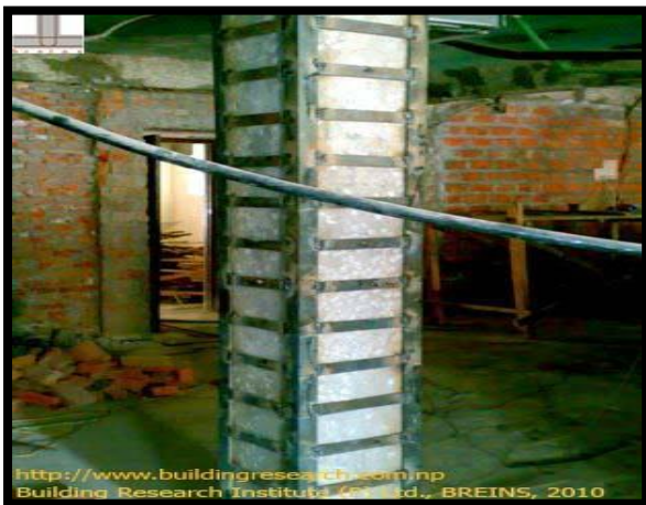
Fig.2.3: A column reinforced with RC jacketing
