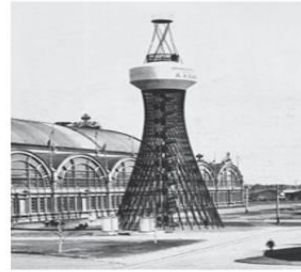
First diagrid tower designed by Vladimir Shukhov in 1896.
