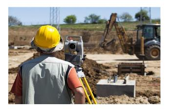
Once the location of the bridge is determined, the main geodetic work will begin, as agreed by various government agencies (architectural, environmental, etc.). The main geodetic works for the construction of bridges include:
