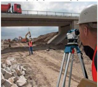
At the next stage, during the construction of the direct bridge, the main geodetic works are: planning of the axes of the centers and supports, planning of intermediate structures, control of the dimensions of the assembly elements supplied from the factory, construction planning and control planning of all parts of the structure, ancillary and temporary structures (buildings, roads, berths, etc.), executive survey of constructed objects, observation of deformations.
