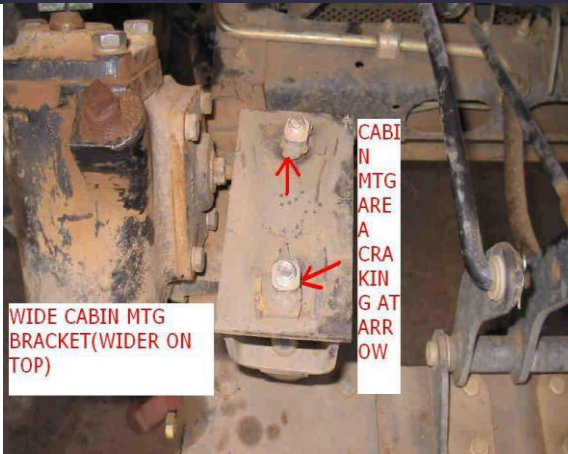
Fig:1.3 shows the complete failure, which is developed on the mounting bracket after traveling 75000 kmph.
